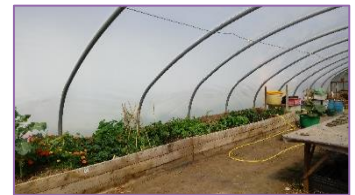
Our beautifully re-sheeted polytunnel
